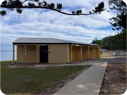
5 Amenities Block & Swimming Pool. Amenities Block is a single storey brick structure with no accessible amenities. The overall layout of the building does not have safety / visibility as a primary concern.
