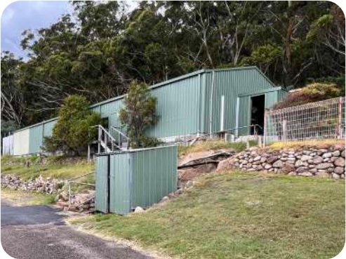
3 Fisheries Facility. Lease for Oyster Operations. Sheet Metal Shed in poor condition and could explore a better, more aesthetic and functional outcome that has a stronger public aesthetic.
