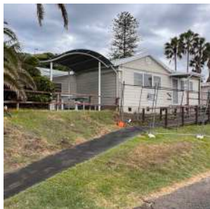
Item 14: Ramp to lower portion of site
