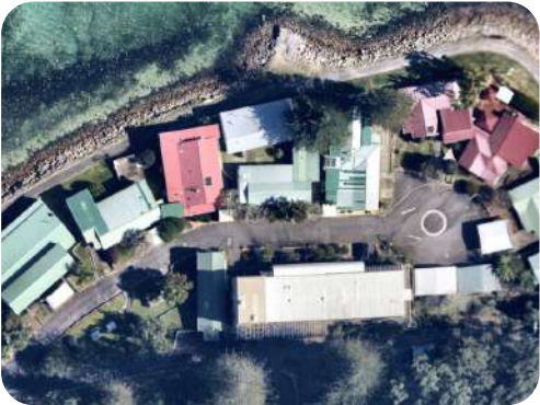
2 The Anchorage (Building 6), The Jetty (Building 7) and the Yachtsman's Rest (Building 10) run against the natural contours of country and they have been subject to water damage and are in general disrepair.
