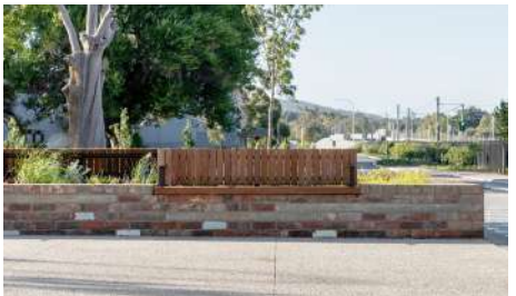
Project: Kelmscott Train Station/SDS
