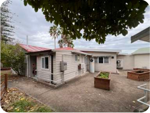
1 Star Fish Lodge (Building 2), Spinnaker Lodge (Building 3) and Mariner's Cottage (Building 4), have seen interstitial links added over time and this has caused clutter in this area of the site and makes it hard to easily navigate through the area.
