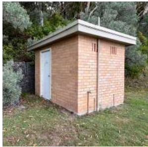
Item 17: Brick Amenities Block
